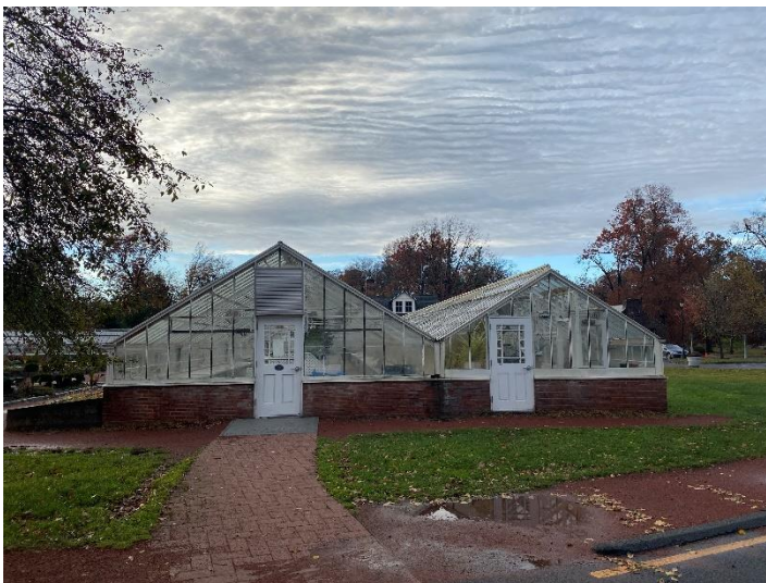
Two of the three greenhouses “before” renovation
